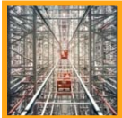
ASRS Warehouse Mechelen, Belgium
