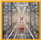
ASRS Warehouse Mechelen, Belgium
